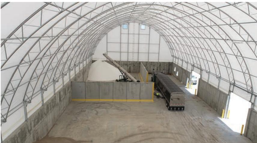
Trusses include upgrade to support the weight of a future hanging fill conveyor.
